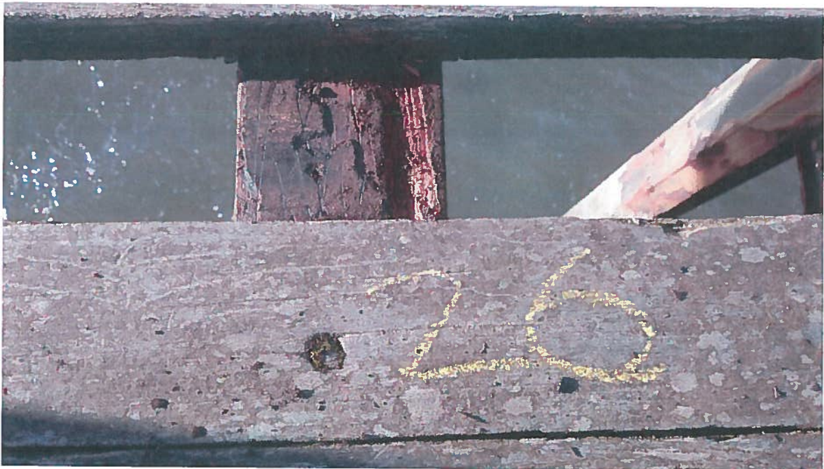
Photo 3 Joist 26 in fair condition. Stress estimated = 0.543
